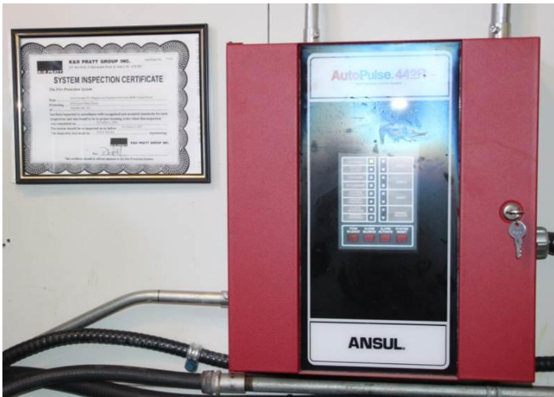
Fig 17. Typical fire detection and extinguishant activation panel.
