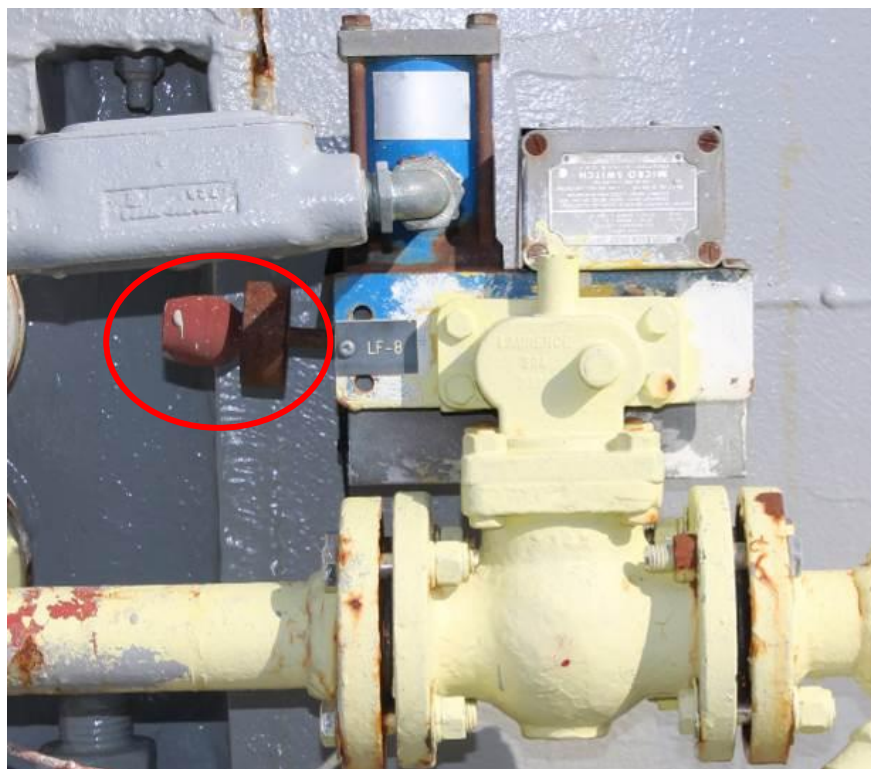
Fig 14. HWD GGA external block valve LF-8 manual activation handle in a position with restricted access.
