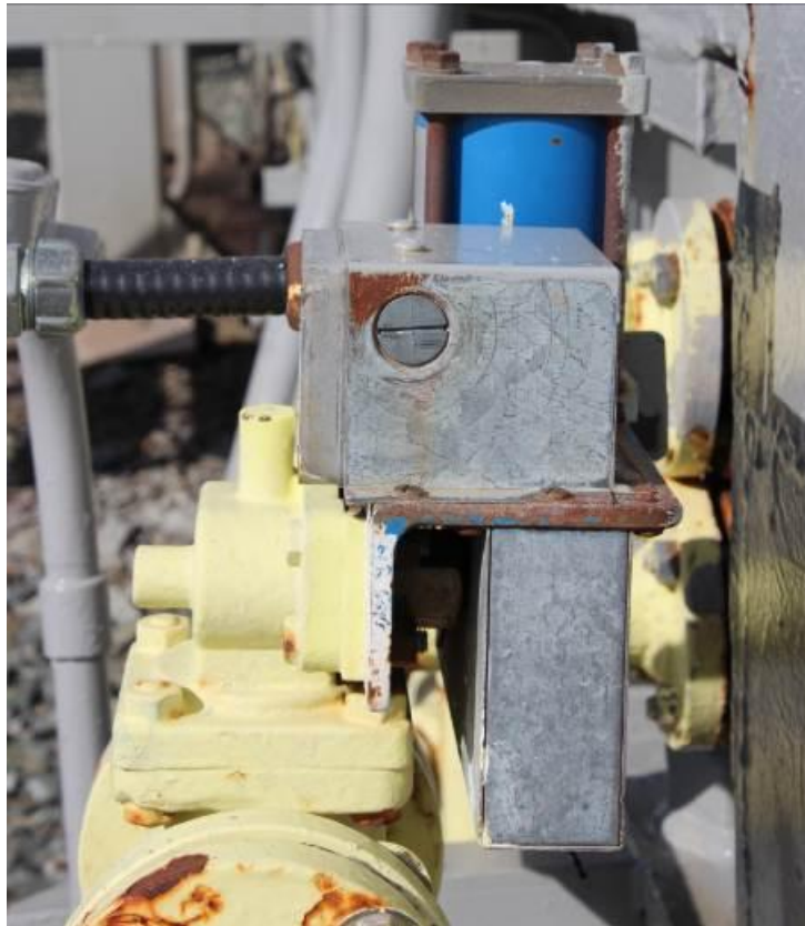
Fig 13. HWD external block valve LF-8 with switch not wired and blanking plug fitted.
