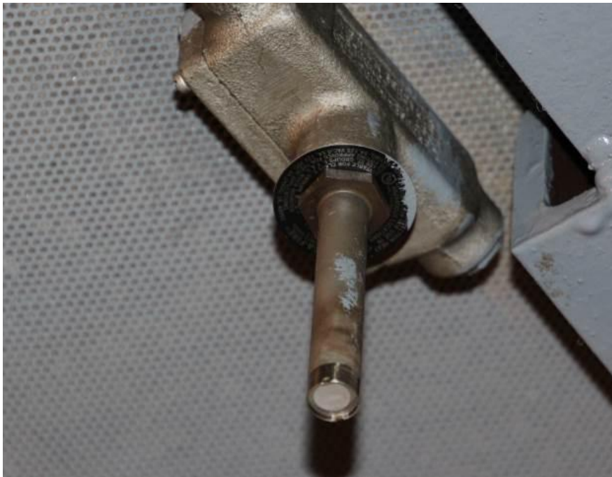
Fig 18. Ceiling mounted fire heat detector.
