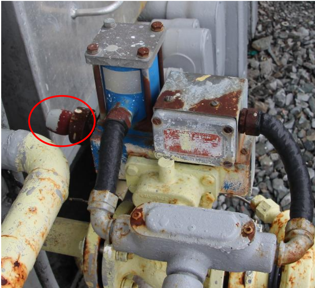
Fig 15. HWD GGB external block valve LF-8 manual activation handle in a position with restricted access.
